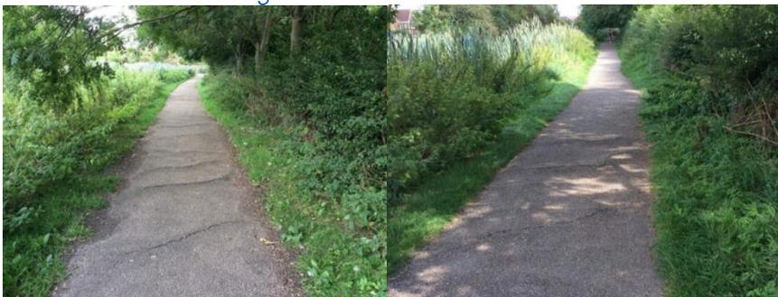
Between Gamston footbridge 6b and lock 3 there are three significant areas of multiple tree root lift damage to the towpath surface, to be repaired by contractors working on behalf of the Trust – delivery by end of March 22.
